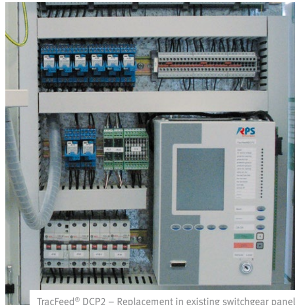
TracFeed® DCP2 – Replacement in existing switchgear panel
