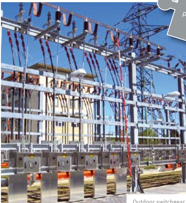
Outdoor switchgear
