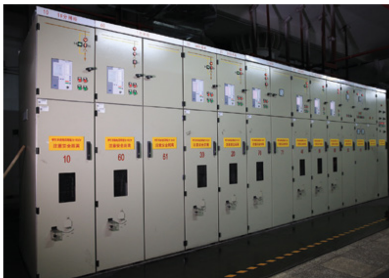
Figure 8: DC switchgear TracFeed® TDB for DC 1,5 kV in a substation of Line 6 in Beijing
