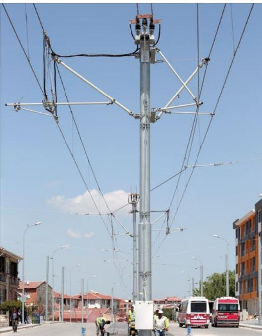
***Mast disconnector with motor drive***
