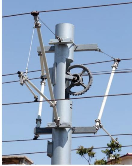
***Semi-integrated tension wheel assembly***
